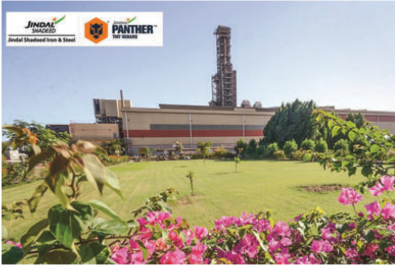
Jindal Shadeed Iron & Steel, Sohar.
